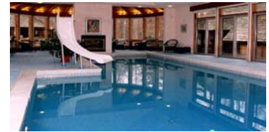
This 18' x 40' indoor concrete pool is a customized shape. The deck is stamped colored concrete.
