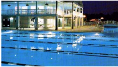
This 9500 square foot gunite concrete pool has a random rectangle shape. The deck is poured concrete. This is the largest community pool in Central Virginia.
